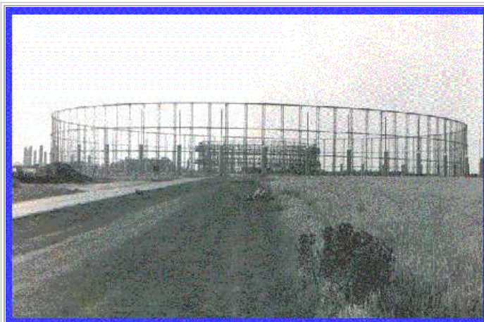
High frequency radio interception antenna (AN/FLR9)
