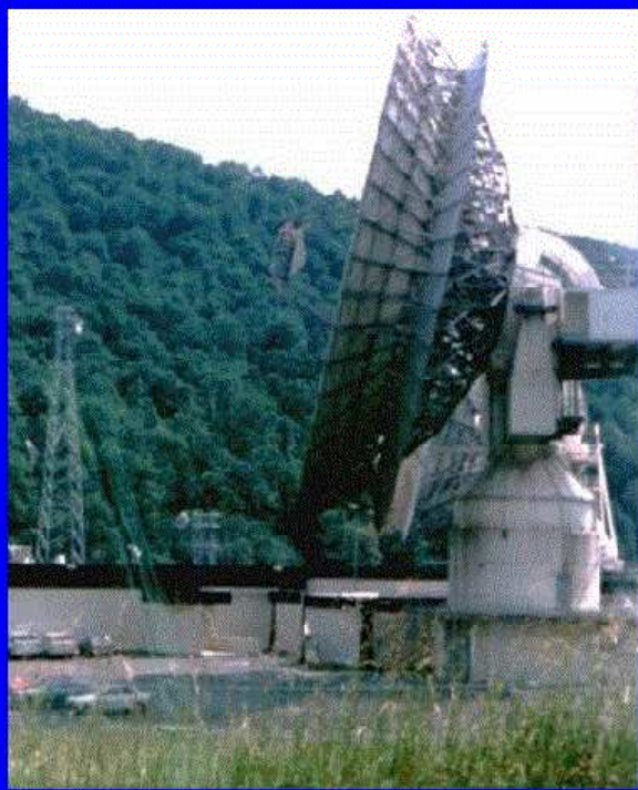
Satellite ground terminal at Etam, West Virginia connecting Europe and the US via Intelsat IV
