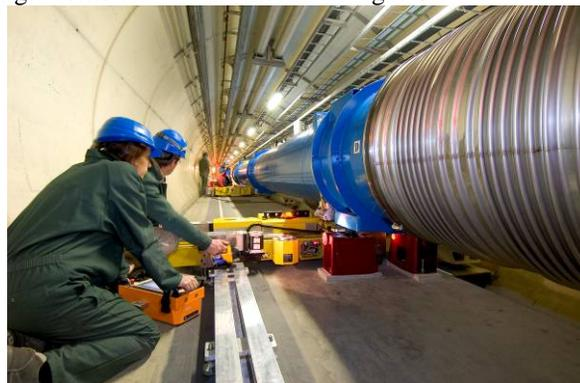
Figure 1: Transfer of a main dipole magnet on the support jacks.
